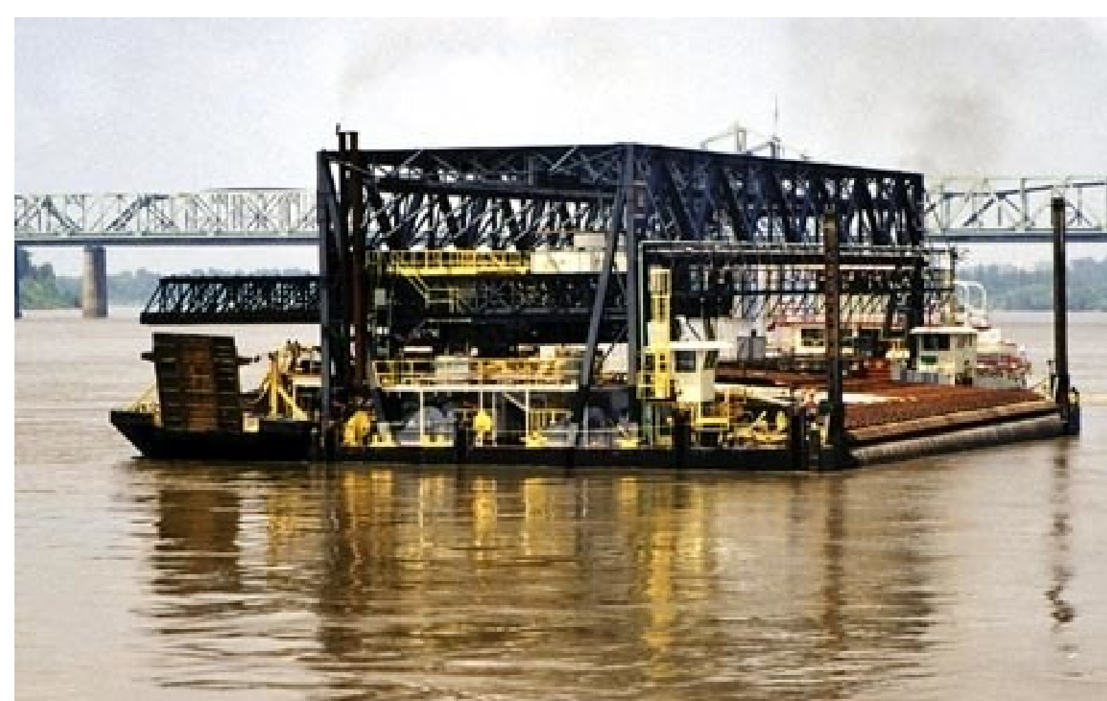
Figure 1. Current Mat Sinking operations
